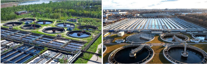
Figure 1. General (panoramic) view of the wastewater treatment plant
