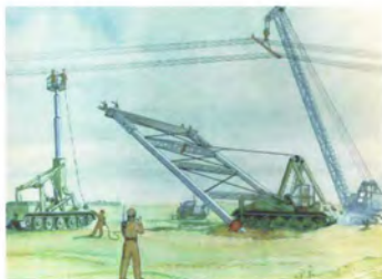
Fig. 14. String tightening on anchor support.
