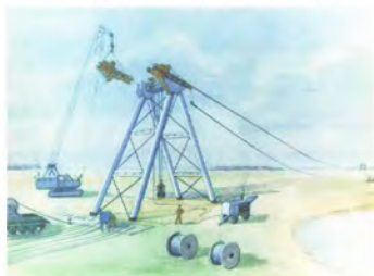
Fig. 16. Technological platform to assemble a string track structure.
