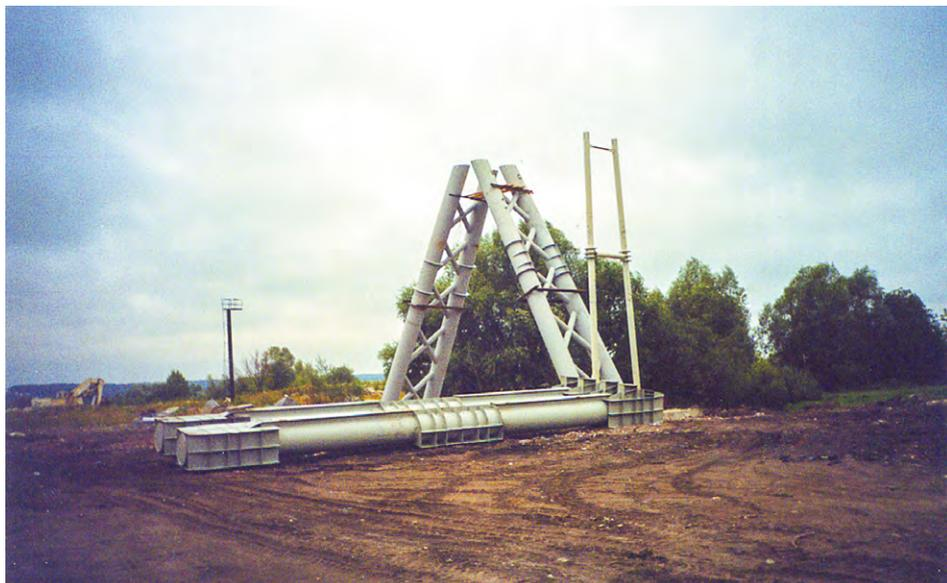
Installation of assemblies for the second anchor support at the UST Track Structure stand under construction. Ozyory, Moscow Region, August 2001
