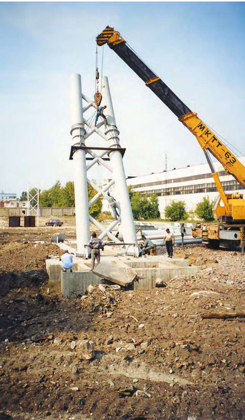
2001. Construction of a string-rail track structure at the string transport test site in Ozyory
