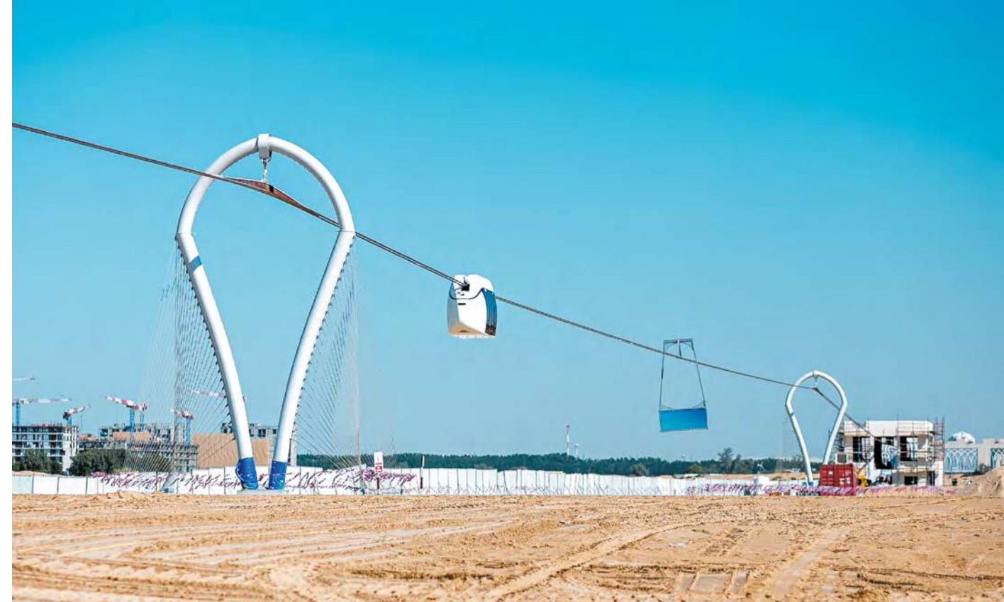
2019. Construction of string track in Sharjah (UAE)
