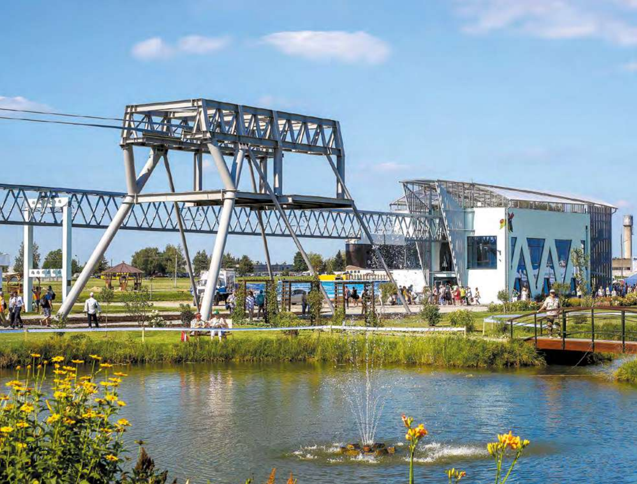
2018. Anchoring structures of string tracks in EcoTechnoPark: one is building-like, the other is steel framed
