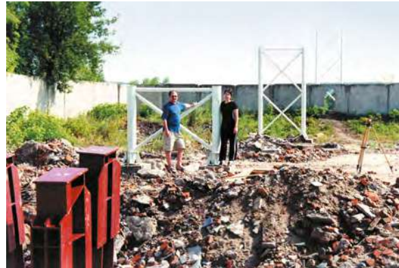
2001. City of Ozyory. Construction of the string transport test site. My wife Nadezhda Kosareva, an employee of my engineering company "Unitsky Scientific Manufacturing Company" is next to me
