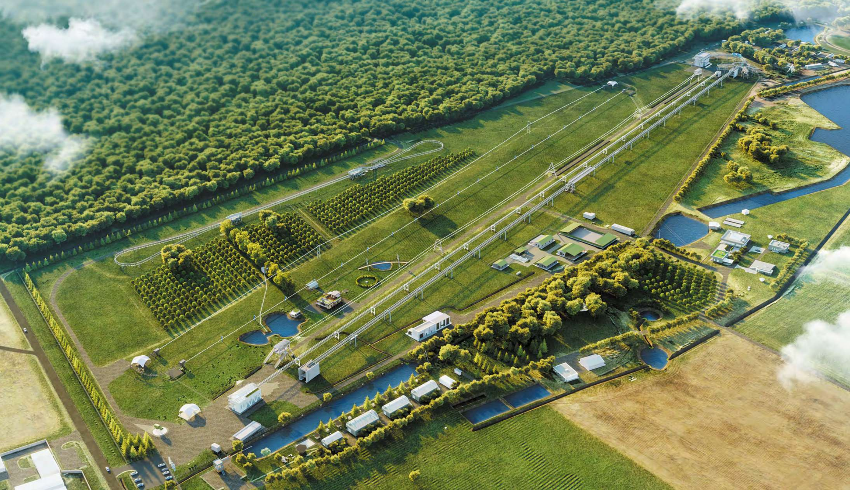
2019–2020. EcoTechnoPark test and demonstration center built on the territory of a former tank range
