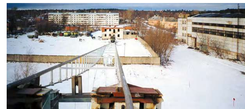
2002. Winter testing of string transport at the Ozyory test site
