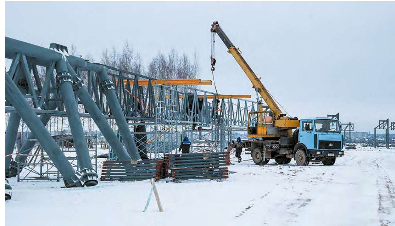
2017. EcoTechnoPark. Construction of a cargo route
