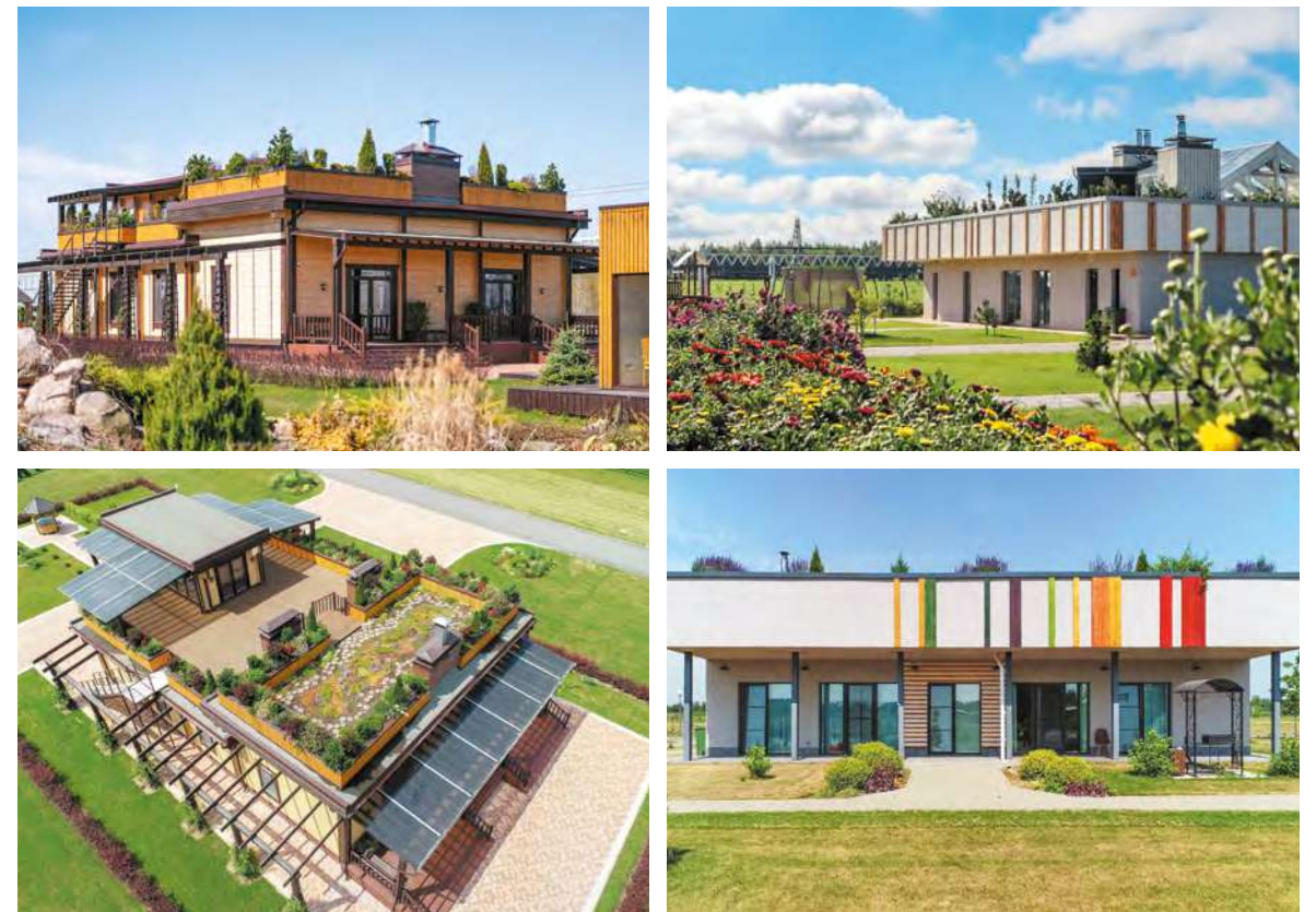
2021. EcoTechnoPark. Ecohouses, during the construction of which green technologies and environmentally friendly materials were used
